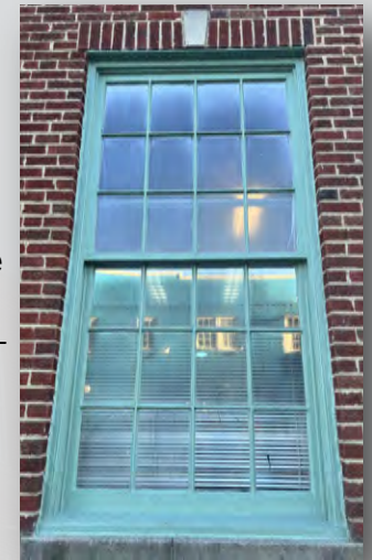
12 over 12 wood window on E. Howell side.
