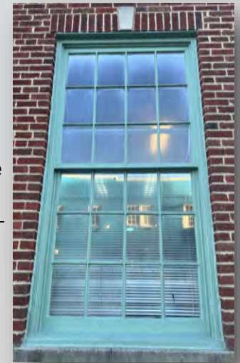
12 over 12 wood window on E. Howell side.
