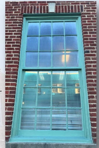
12 over 12 wood window on E. Howell side.
