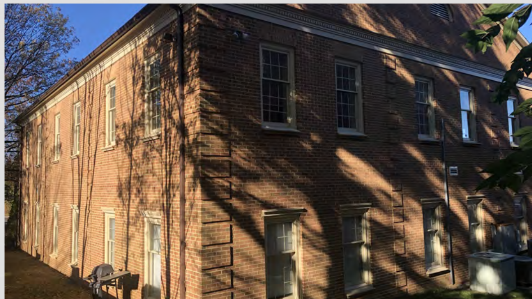
Rear of Building
